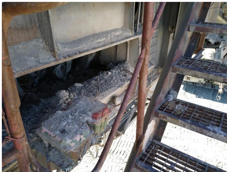
Figure 3. Entrance to the chamber.
