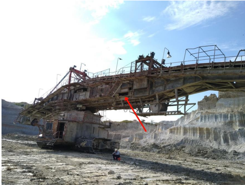
Figure 2. Opening of the chamber of the propulsion part intended for lifting the break part of the unloading lane.
